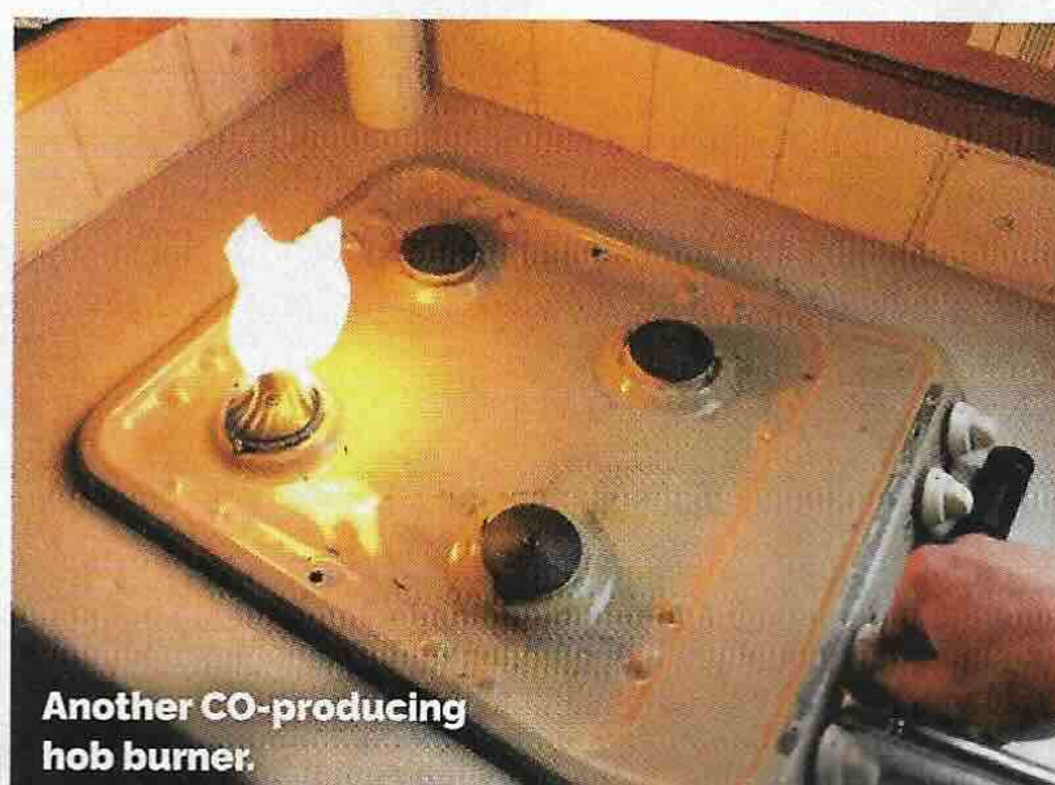
This hob was in good operational condition except that spiders had moved in to the front left burner over winter, causing it to become dangerous.
