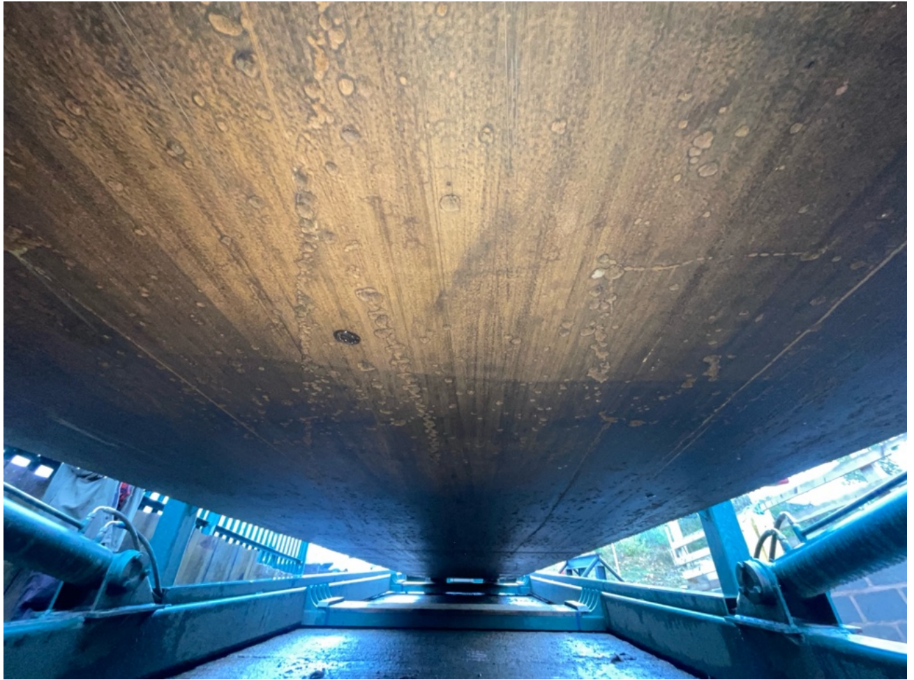
Longer view of the base plating showing the pitting arrested. Note a single graze exists to the right hand of the photo, otherwise the paint has resisted damage. This is a continuous cruiser, paint 5 years old at time of survey.
